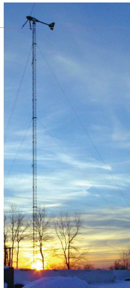
AT LEAST one acre of open land and an adequate wind resource are necessary for a small wind installation.
