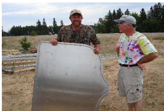
Pictured here is David Winkelman of Winkelman's Environmentally Responsible Construction (WERC) holding the tail vane section of the wind turbine with Bob McLean of HUG observing the giant "erector set" project taking shape
