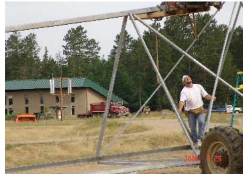
Foreground is the start of the 120-foot tower that will hold the 20-kilowatt Jacobs wind turbine. Back ground is the small wind turbine test pole with 3 turbines and a weather station mounted on it. Behind that is the HUG campus main office, made from straw bales and earth plaster.
