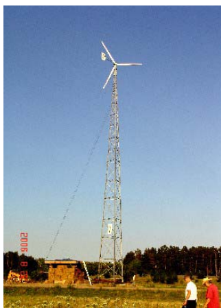
Here the tower is almost in place.
