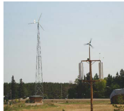
Shown here is the Jacobs wind turbine-producing energy. In the foreground is the small wind turbine test pole, which has two experimental vertical wind turbines that seem to always be turning and flashing in the sun. It has a 0.5-kilowatt bladed turbine for comparison. It has a weather station that measures wind speed and direction and rain fall. It is loaded with instrumentation, measuring all the performance details and making the data available on the web.
