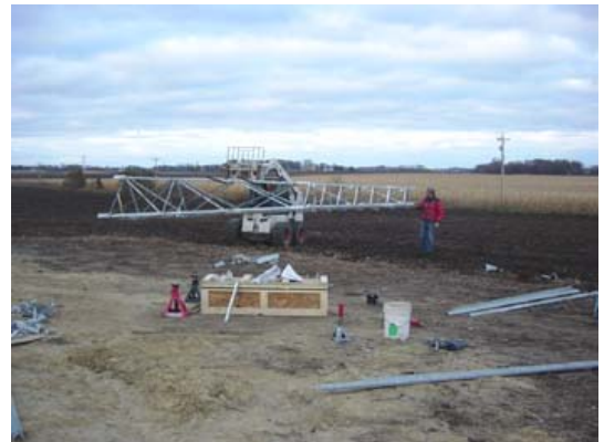
Tower starting to take shape.
