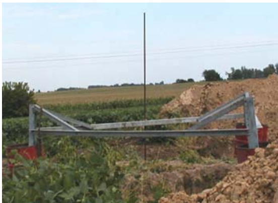
Wind turbine tower foundation ready for pouring concrete.
