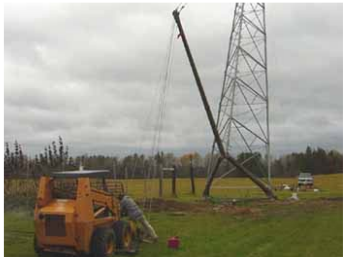
Tower almost in place.
