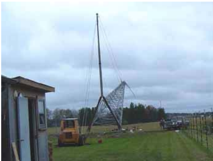
Gin pole shown during tip-up
