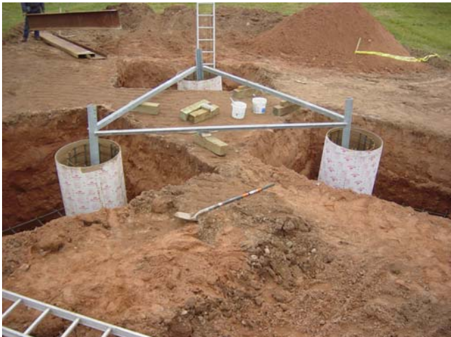
View of pier foundation being set up for.
