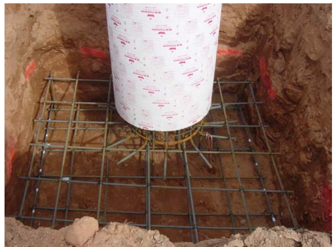
View of base of pier foundation
