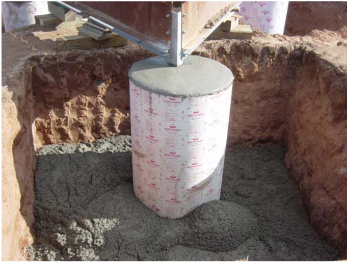
Concrete pouring of foundation
