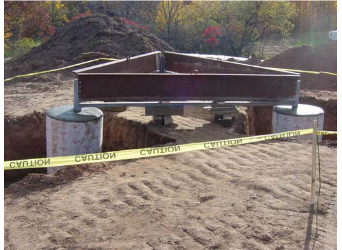
Pier foundation with template in place.
